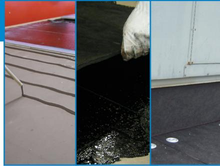
Adhere SOPRASmart system with mechanical fasteners, DUOTACK 365 insulation adhesive, or hot asphalt.
