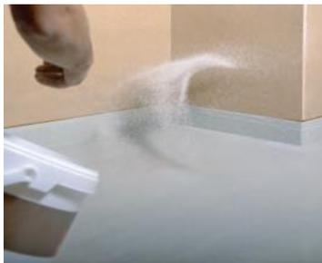
Note: Broadcast aggregate must be properly sealed with ALSAN RS Finish. Prior to applying finish seal coat, remove excess aggregate from surface by broom, vacuum or oil-free blower. See ALSAN RS Finish Application Guidelines for information regarding application of ALSAN RS Finish and surfacing components.
