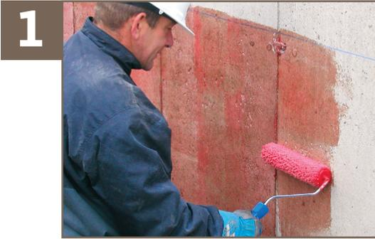
1 Prime the substrate with ELASTOCOL Stick, ELASTOCOL Stick Zero or ELASTOCOL Stick H<sub>2</sub>O.
