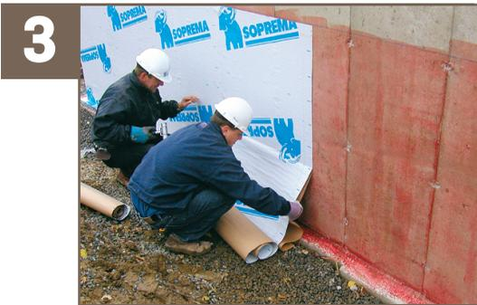
3 Gradually peel back the remaining silicone release film, making sure the membrane is completely adhered.
