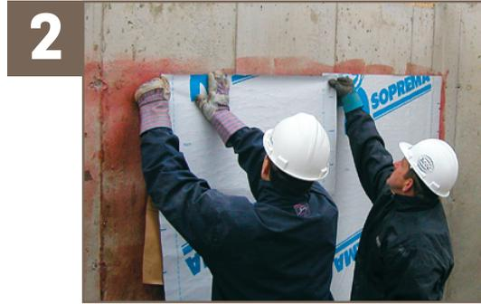
2 Peel back the top part of the silicone release film. Adhere COLPHENE 3000 to the substrate, making sure the membrane is well aligned.
