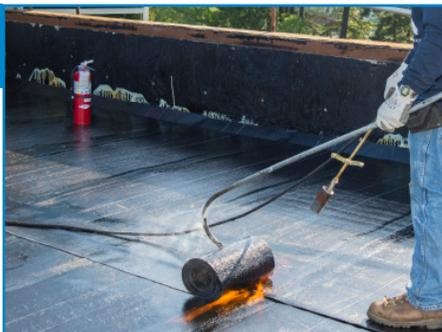
Roll self-adhered portion of Duo Selvedge side lap and then heat weld remaining 60%. Apply SOPRALAP cover strip over all end laps.
