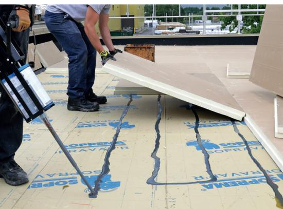
SOPRA-ISO is a rigid polyisocyanurate thermal insulation panel for use in approved multi-ply membrane and flashing assemblies. SOPRA-ISO is composed of closed cell polyisocyanurate foam bonded to fiber reinforced/organic mat facers on the top and underside. With one of the highest R-values among all types of insulation (R-5.7 per inch), SOPRA-ISO forms a roof system that is slimmer, yet more effective.
