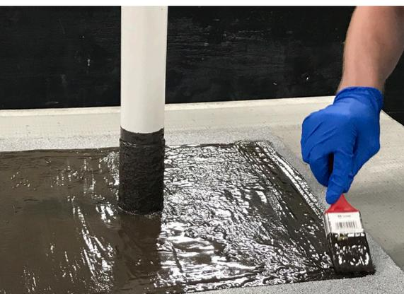
ALSAN Flashing is a unique polyurethane bituminous resin specifically formulated for liquid-applied flashings, other details and maintenance applications. ALSAN Flashing utilizes a reinforcement that, in combination with its unique chemistry, provides an extremely durable and easy to apply flashing solution. The variety of suitable substrates, including concrete, masonry, wood, metal, PVC pipe and SBS granule and sand surfaced sheets, make ALSAN Flashing extremely versatile.
