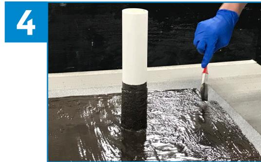
4 Once cured, apply a final coating of ALSAN Flashing at a rate of two gallons per 100 ft<sup>2</sup> to the pipe and field, extending approximately 1" past the previous coat.
