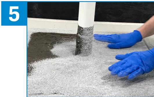
5 While it is not required, if desired, granules may be broadcast into the final coat of ALSAN Flashing to match the cap sheet.
