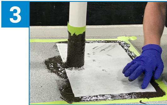
3 Apply ALSAN Flashing to the taped off field area at a rate of two gallons per 100 ft<sup>2</sup>, lay fleece into the first coat and apply second coating of ALSAN Flashing. Remove the tape.
