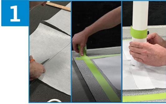
1 Pre-cut the ALSAN Flashing fleece to conform with SOPREMA published details, tape off the area using masking tape and dry fit fleece to ensure proper sizing.
