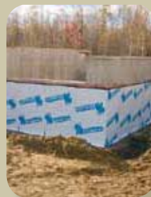
COLPHENE 3000 Self-adhesive membrane for foundation waterproofing
